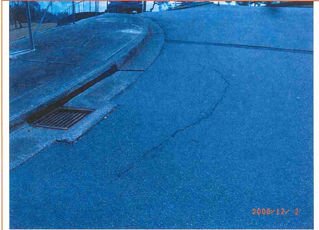
Photo 1 - Longitudinal crack around drainage inlet pit
