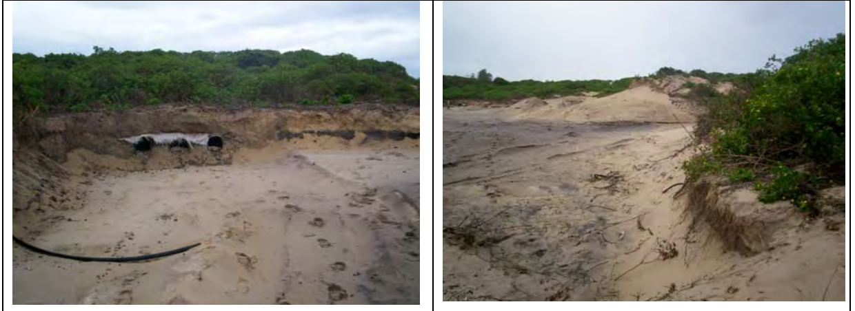
Photo 6 Excavations at RAC8A showing existing subsoil drainage system (21/05/09)
