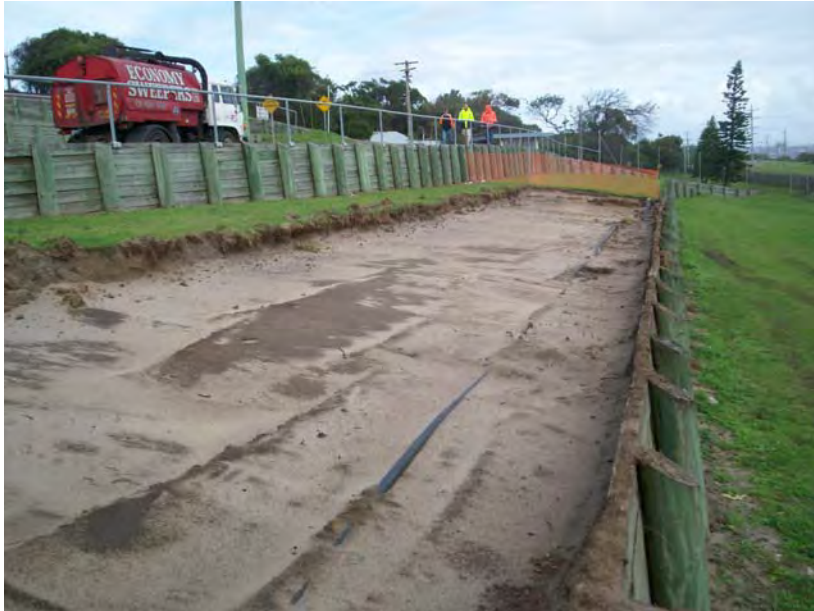
Photo 3 Excavated surface between retaining walls RAC5 (21/05/09)
