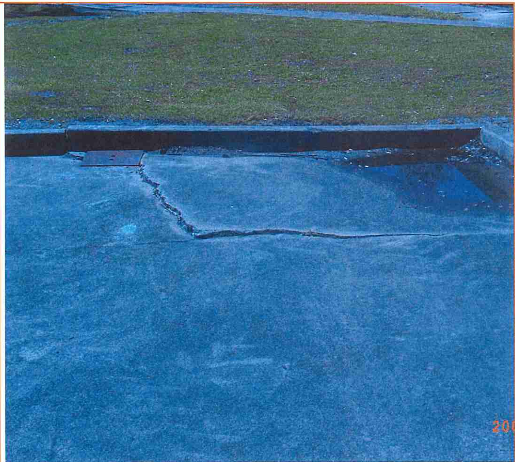
Photo 6 - Crack in concrete slab
